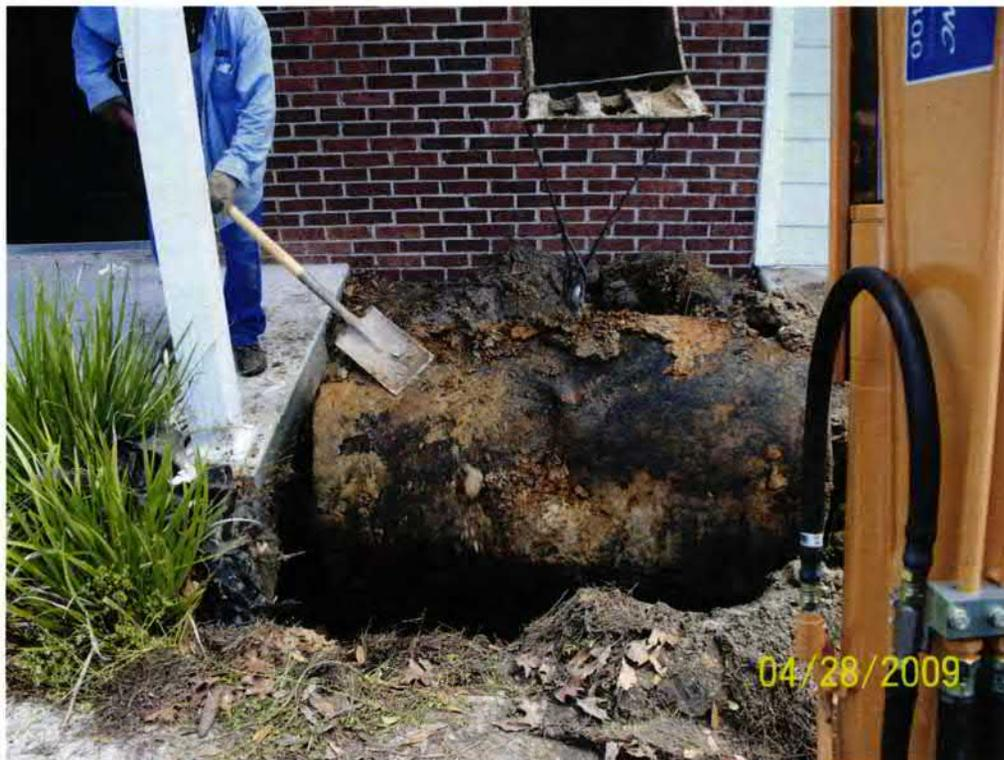
Picture 2: UST 289Birch being removed from the excavation.
